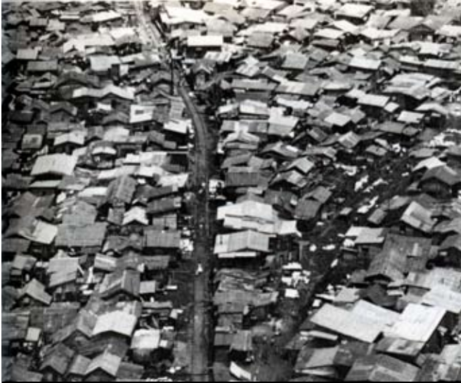
Informal housing built on both sides of a railway line in North Harbour, Manila, Philippines Image reproduced from Juppenlatz, M. (1970). Cities in Transformation: The Urban Squatter Problem of the Developing World . Pg 111 All rights reserved, University of Queensland Press, 1970
