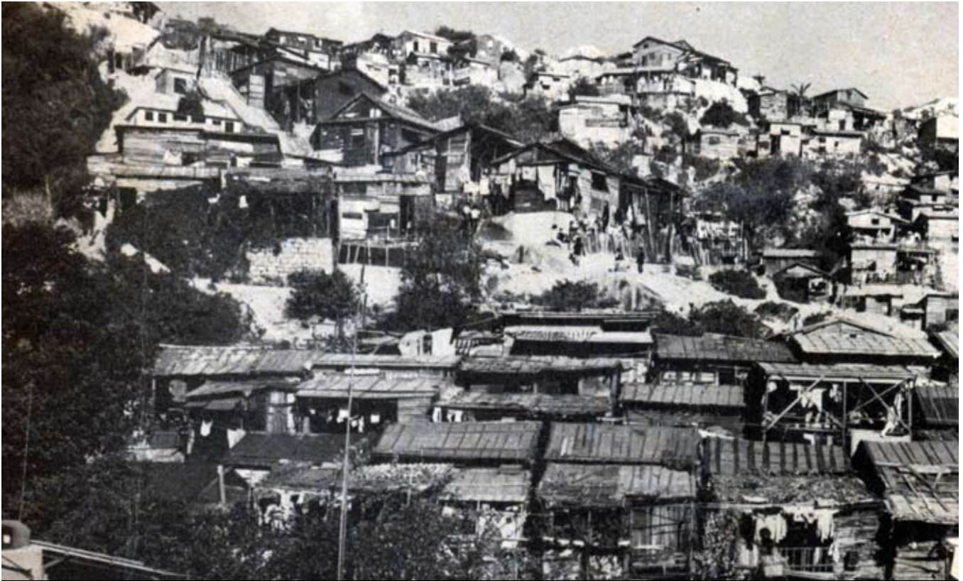
Informal housing built on hillsides in Hong Kong Image reproduced from Dwyer, D. J. (1975). People and Housing in Third World Cities: Perspectives on the Problem of Spontaneous Settlements . Plate 8 between pg 36 and 37 All rights reserved, Longman, 1975
